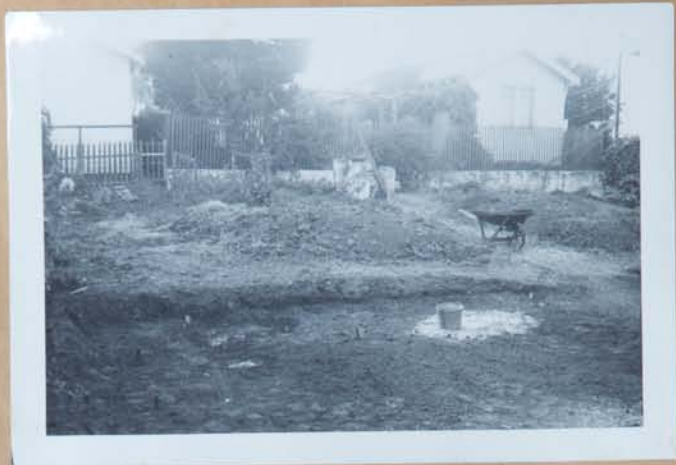
This shows material removed from Patio Area, and is the material - where "Shekey" played the leading role.
