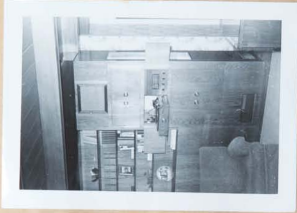
At Top - 12" speaker - next - space for Records; next - Tuner and record changer, Next Television - area - if it when. Amplifier located at bottom. A speaker in each room, Tuner can be turned on or off from each room, but no station selection except at set. At bottom Cold air in take for furnace.
