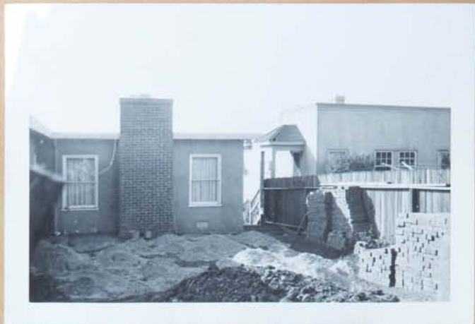
Material for Patio - 5 yards Sand - 3000 Bricks.
