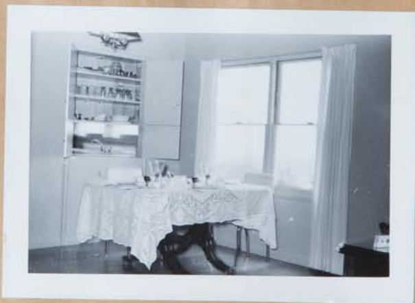
Showing Cabinet which also opens to Kitchen. Pass-through below shelves can be seen.
