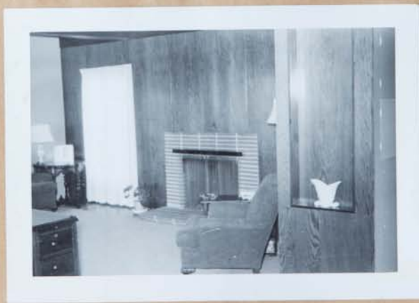
Fire place from Dining Area. All panels glued - practically no nails used.
