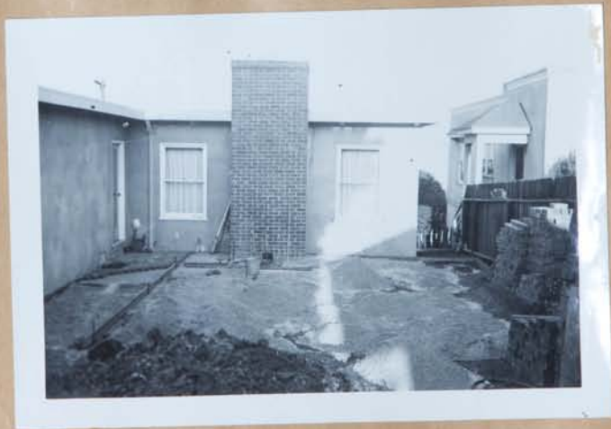
Patio - in course of construction. About - Sept, 1, 1952.
