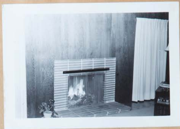
The few interior pictures - which follow - by flash. Fire place - wall - Redwood - natural finish.
